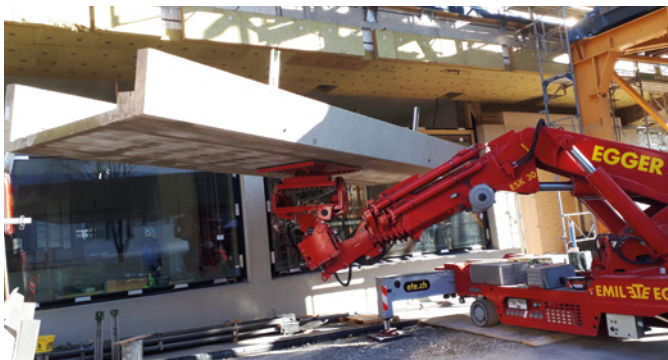
ESK 30: \curvearrowright 2.5 t @ 0.9 m, h = 650 mm; \dashrightarrow 5 t @ 0.78 m, h = 243 mm; \dashrightarrow 2.5 t @ 3.28 m, h = 243 mm; 25 t Montagebock ESK 75: 5 t Montageplatte
